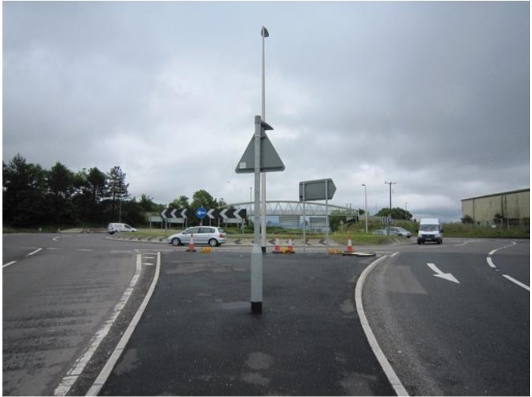
View from west (Services area)
