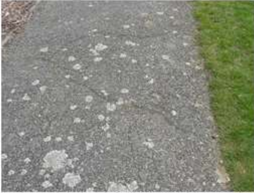
displaced tarmac adjacent to Araucaria Araucana tree
