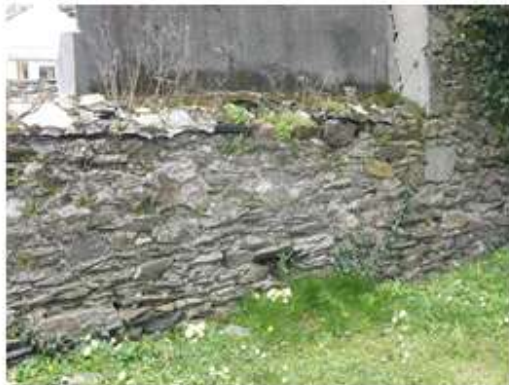
wall between Victoria Gardens and Malvern House
