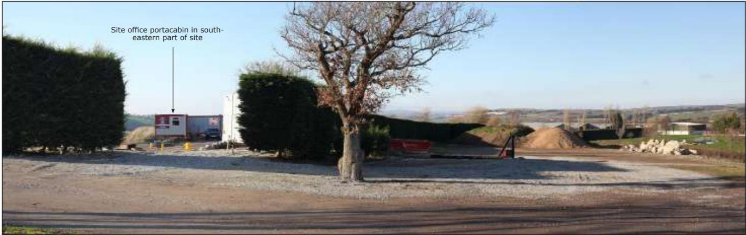
CA8:View from eastern section of PRow (footpath ref 636/3/1) - near the site
