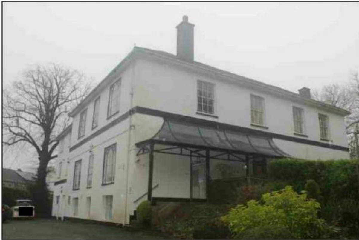
Plate 1: View of west and north elevations, looking southeast
